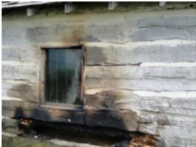
In late May an arsonist set our log cabin on fire. The window, wooden shutters and several logs were damaged.
